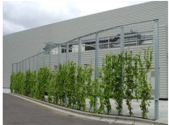
Zaštitno zelenilo u poduzetničkoj zoni Engleska Curtain Green Wall, MMA Design green-walls.co.uk
